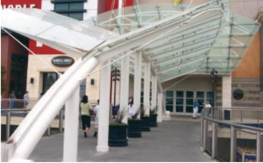
then raised up along its edges. Constructed using a series of king-post trusses assembled from wide-flange steel top chords, HSS compression struts, tension rods, and steel rod bracing, the undulating roof bears lightly on a diagonal HSS truss framing the clerestory glass.
